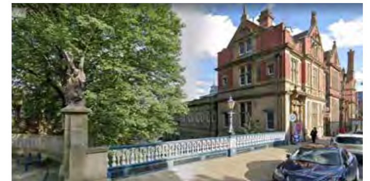
10 Trinity Street - View East
