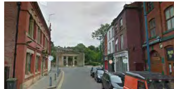
6 Market Street - View East
