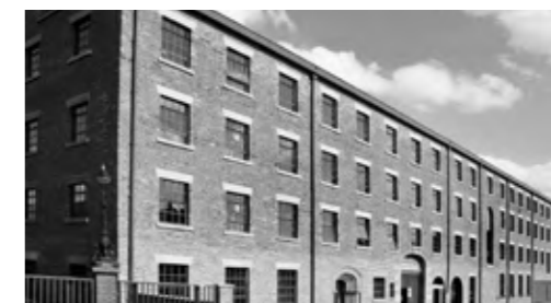
H Castle Street Mills | Grade 2 Listing | Former Cotton Mill. 1805 / Renovated 2009
