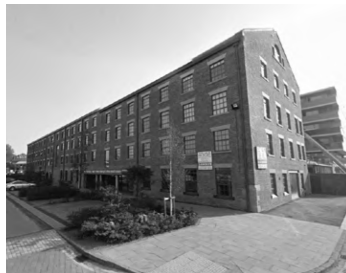
Castle Street Mills Redevelopment by Urban Splash
