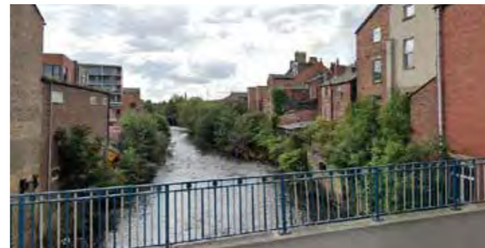
2 Melbourne Street Bridge - View West
