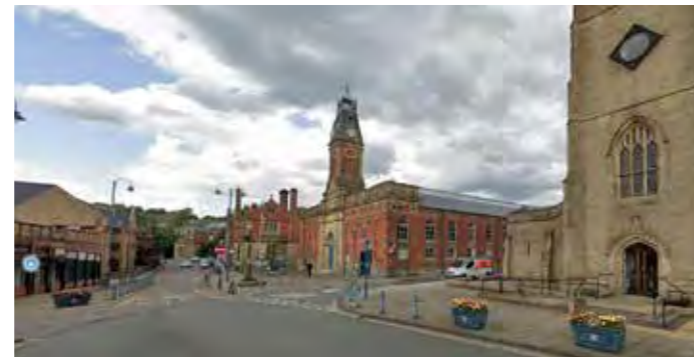
1 Armentieres Square - View North
